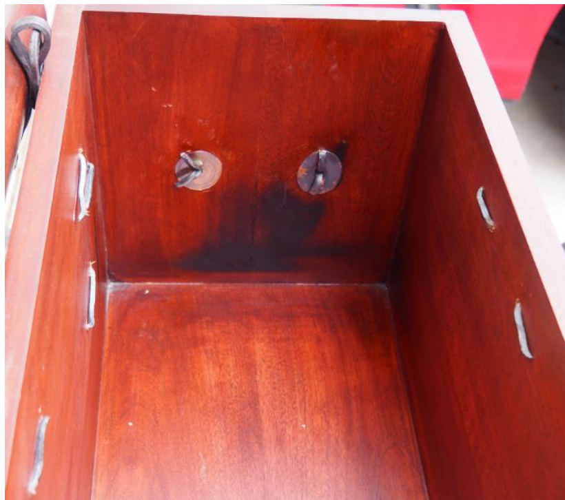
Figure 14 Nails in my box bent over and cinched
